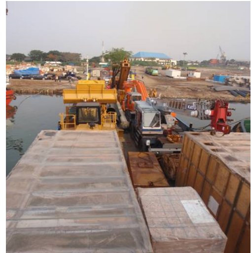
Fully loaded condition
